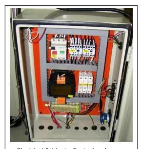
Electrical Cabinet –Control and accessory power transformer, circuit breakers and main disconnect.
